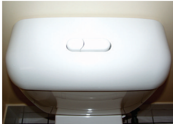
Dual-flush toilets like this one are common in Australia. The left button saves water by flushing down liquids with a 0.6-gallon flush, while the right button flushes solids with a 2-gallon flush.
