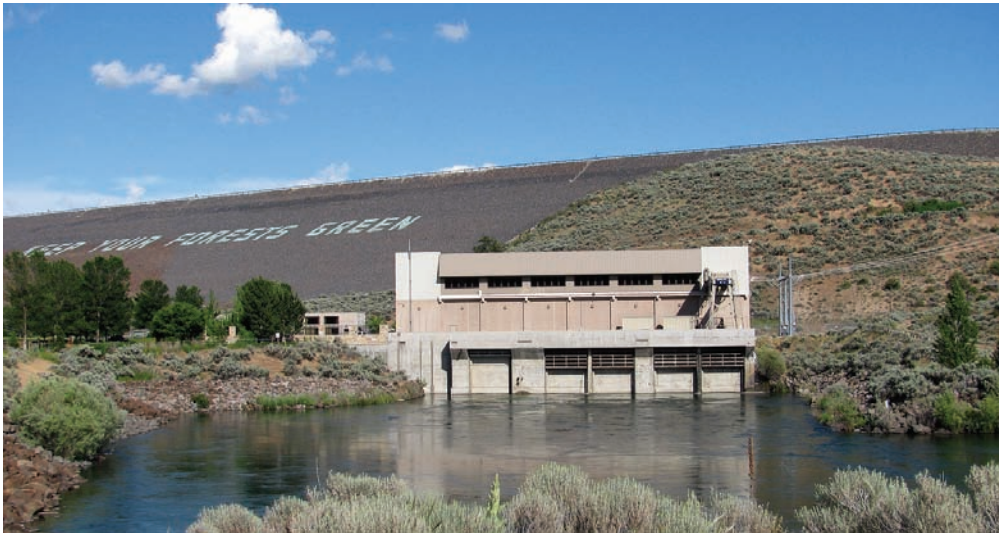
The Lucky Peak Power Plant in Idaho collects energy from the Boise River as it flows through a dam.
