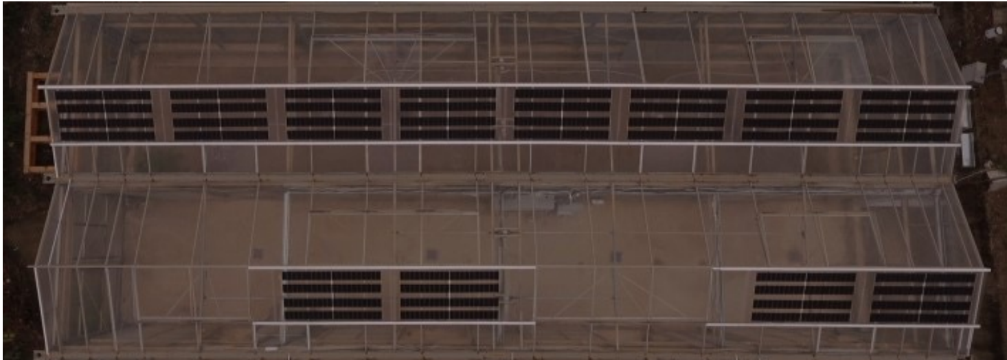
Photovoltaics from the outside
