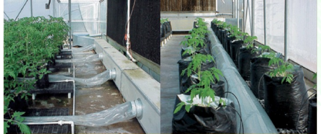
Plastic perforated pipes placed at ground level
